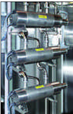
Triple Quattrra 100 UV system configured to provide more exposure to the UV light, ensuring a higher kill rate of the bacteria.
