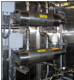
Dual Quattrra 50 UV system configured to provide more exposure to the UV light, ensuring a higher kill rate of the bacteria.
