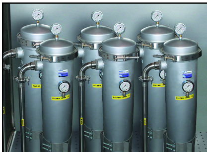
Filters configured to remove particulate matter that may inhibit the effectiveness of the UV system.
