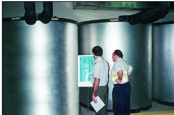
Two 1,600 gal. Ice Storage Tanks
