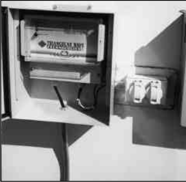
Triangular Wave Technologies, Inc. Microprocessor TWT-5C8-404 installed in a weatherproof electrical box on the outside wall of the building.
