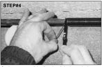
Continue to wrap until the 4" section of pipe is completely covered. Fasten down the end of the coil with the second cable tie (provided). You can hold the first layer in place with cloth tape or electrician's tape.
