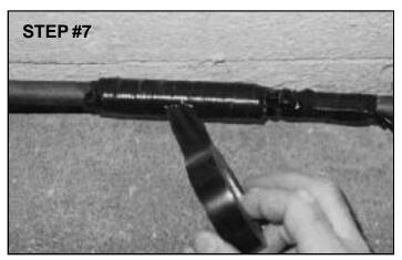
Wrap the coil with electrician's tape or cloth tape (duct tape) to help maintain a tight coil and protect the coil from being disturbed.
