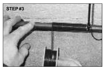
Wrap the signal wire around the pipe in a tight coil, in a clockwise manner, so that the adjacent wires are touching each other.
