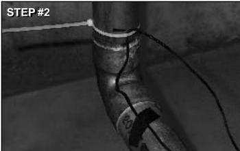
Fasten the signal wire to the pipe with a cable tie (provided) at one end of the 7" section.
