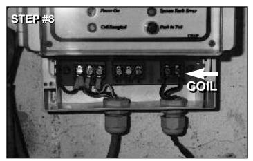
Guide both wires to the Triangular Wave Unit and leave about 2" of extra wire.
