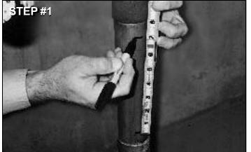
Measure and mark a 7" section in the middle of a straight pipe segment.
