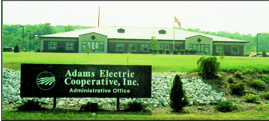
Adams Electric Cooperative, Inc. Headquarters Building
