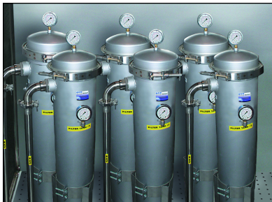
Four stage filtration configured to remove particulate matter that may inhibit the effectiveness of the UV system.
