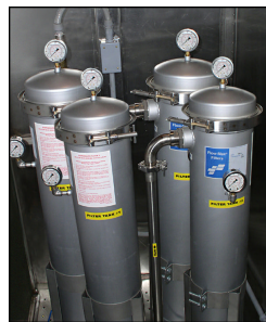
Two stage filtration configured to remove particulate matter that may inhibit the effectiveness of the UV system.
