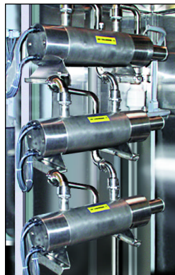
Triple Quattra 100 UV system configured to provide more exposure to the UV light, ensuring a higher kill rate of the bacteria.
